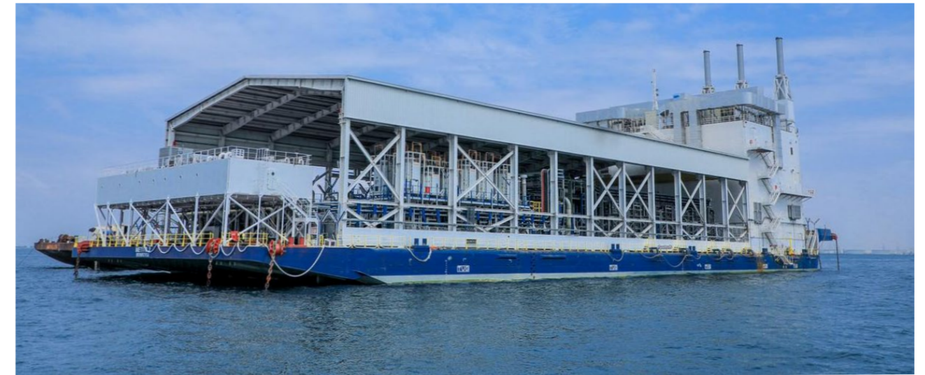
Saline Water Conversion Floating Plant, Saline Water Conversion Corporation
