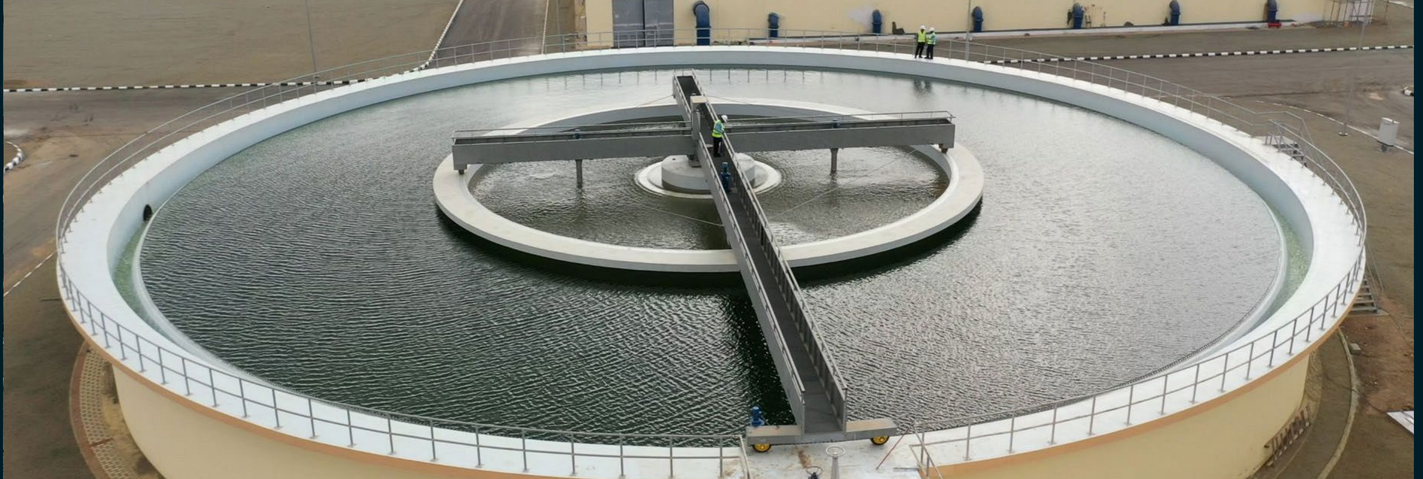
Sedimentation tank in wastewater treatment plant, National Water Company
